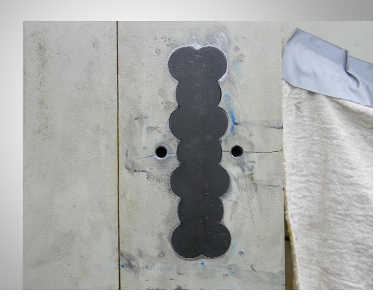
Using C4 Castmaster stitching pins to repair the crack.
