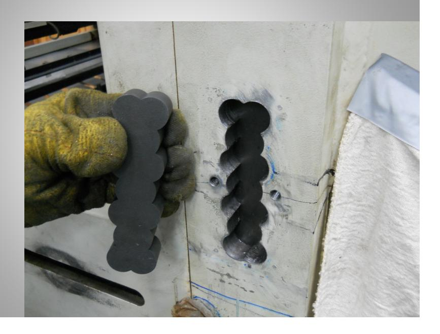
L60 lock installed and ready to have the crack stitched and hand finished.
