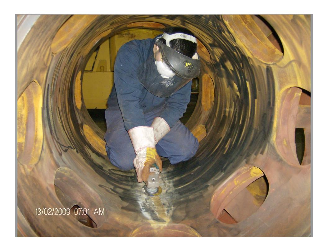
Inner bore of cylinder machined and ready to accept new sleeve.
