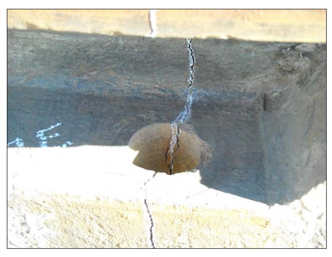
Metal stitched 1E using (1) C4C stitching pin and (1) C3C stitching pin.
