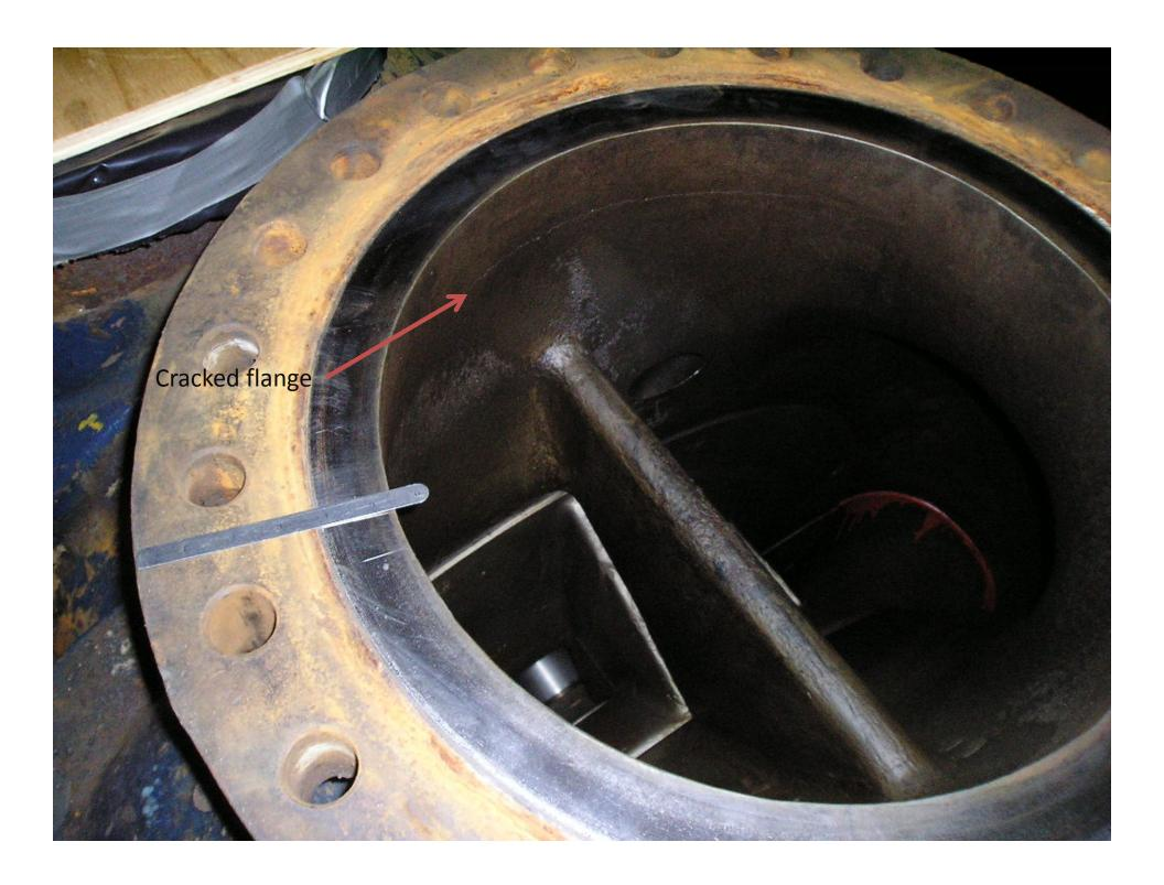
Removing cracked flange so the new manufactured flange can metal stitched into place
