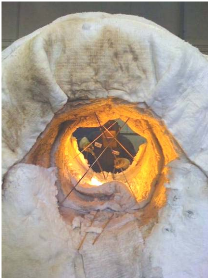
Brazing to fill the groove
