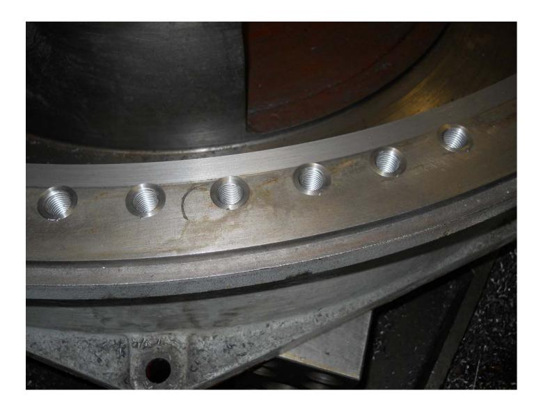
7. Stitching required inside the radius area where a low spot occurred when machining new sleeve. First Row of holes was drilled to receive L8 stitching pins.
