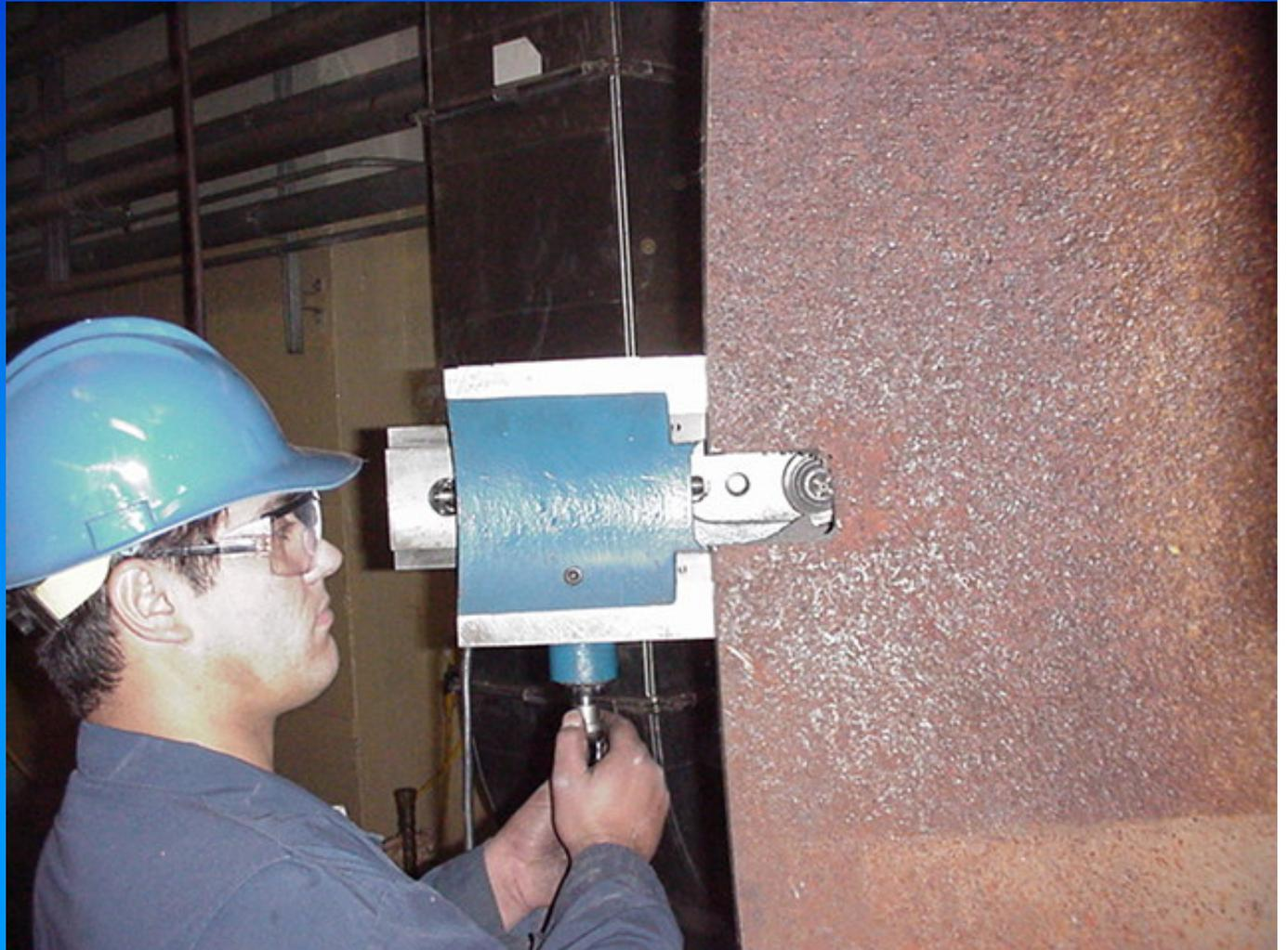
The slots were created to accept steel locking-lugs welded to the new steel flange
