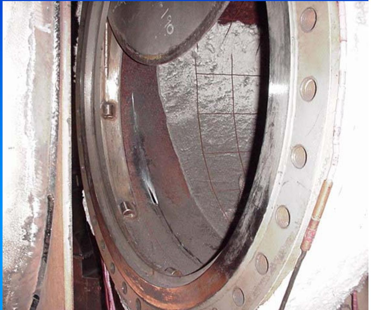
Repairing the damage in place could only be done by replacing the damaged flange and port wall
