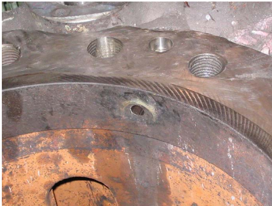
The water hole repair is completed
