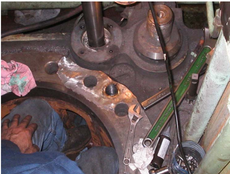
Stitching continues until the repair is complete.
