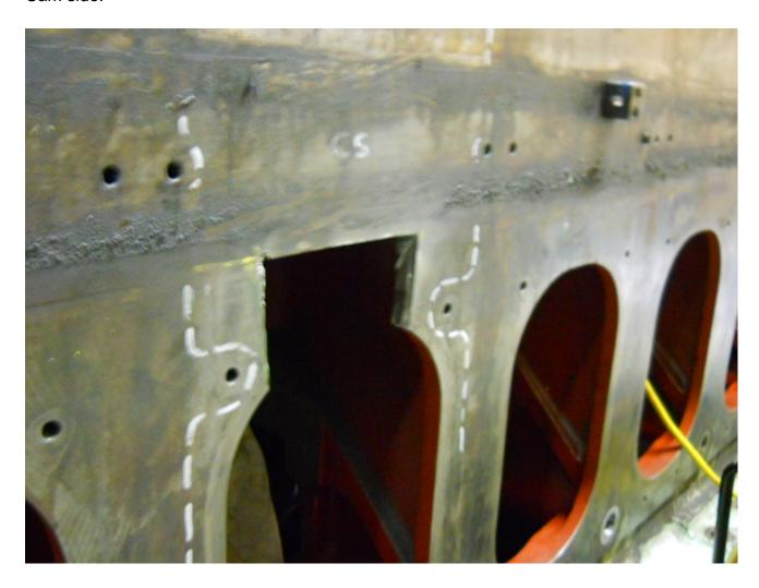
New casting fit in place and stitched with C3 Castmaster pins.
