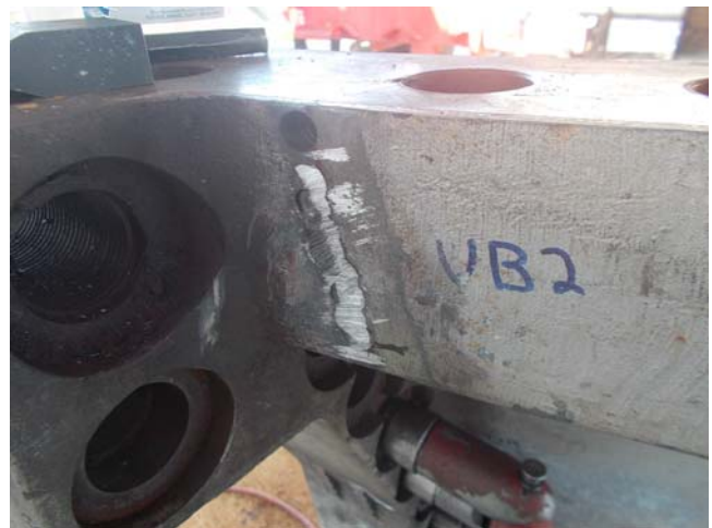
Metal stitching in process
