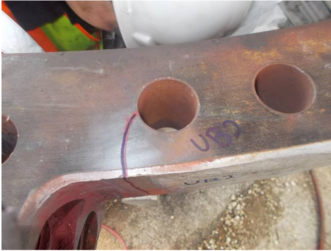
#3 Bolt hole on B side of upper shell flange
