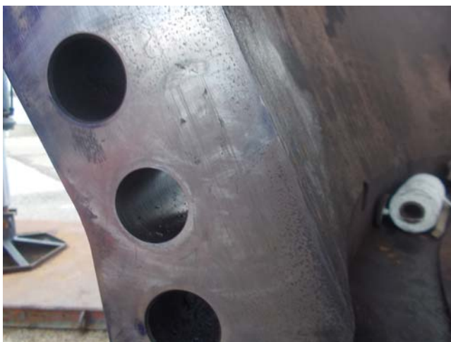
Completed repair after finish work
