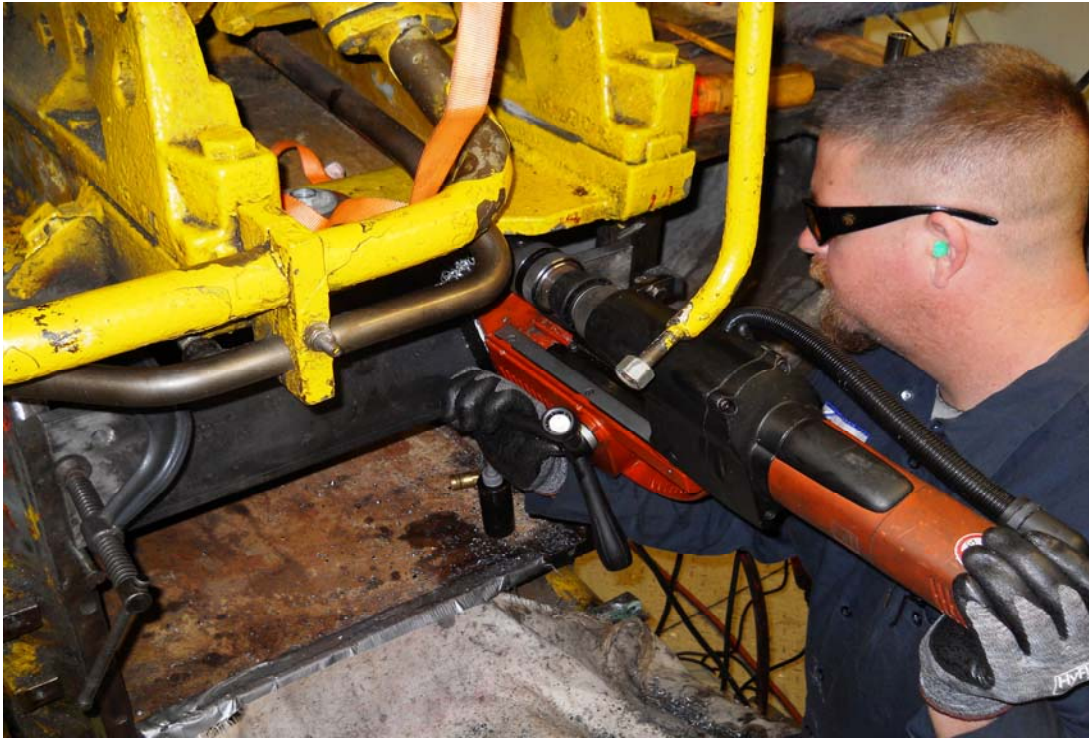
#6 Installed Full-Torque thread inserts.
