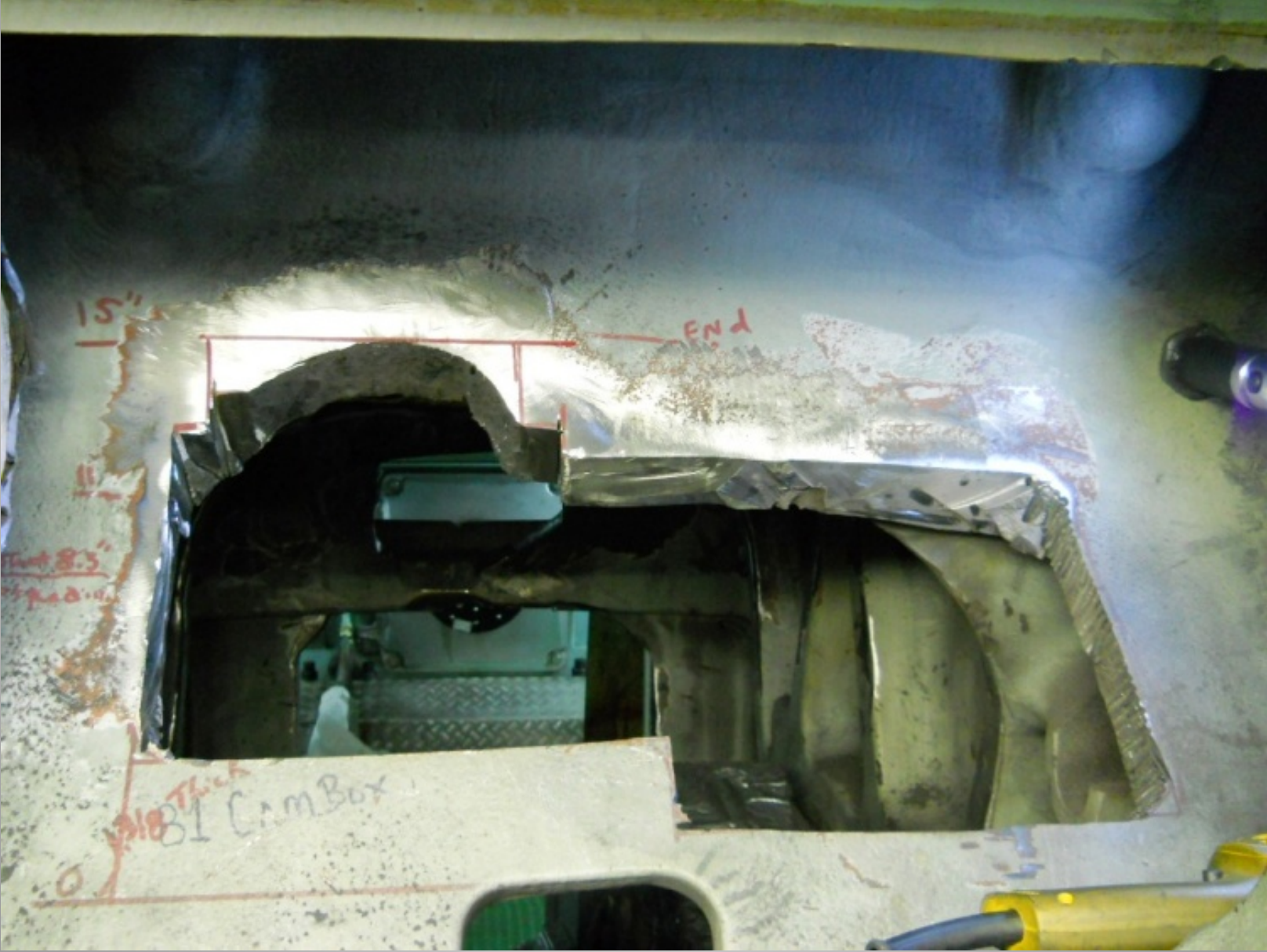
Damaged area cut out and ready to accept patch
