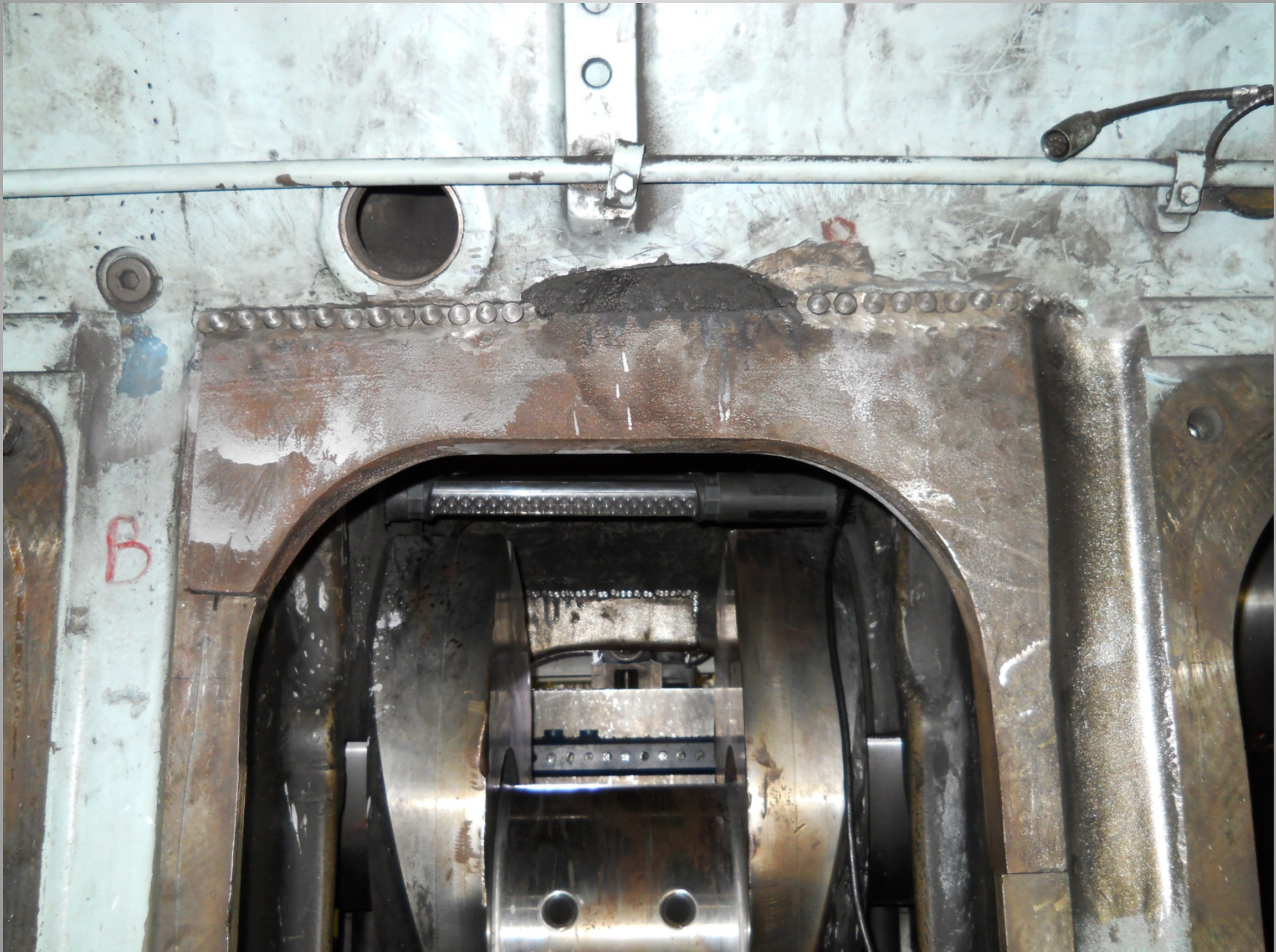
Metal stitching in process on the B side Inspection Door Gasket Surface
