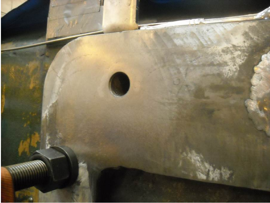
Stitching completed ready for insert to be installed.
