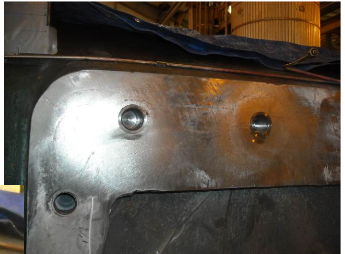
FULL-TORQUE insert Installed.
