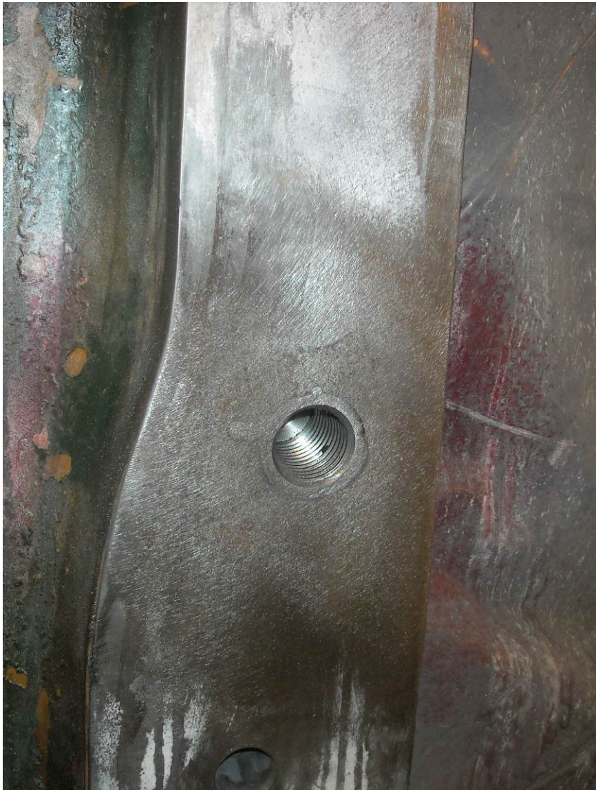
Completed repair after installation of the FULL-TORQUE FFB-12 insert.
