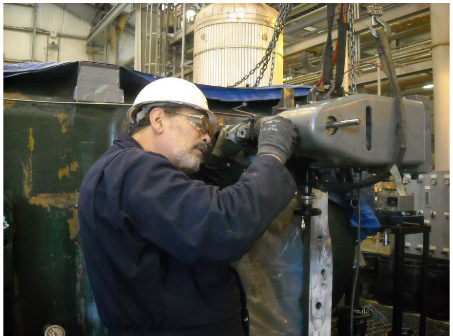
Setting up the portable mill to machine flat for gasket seal.
