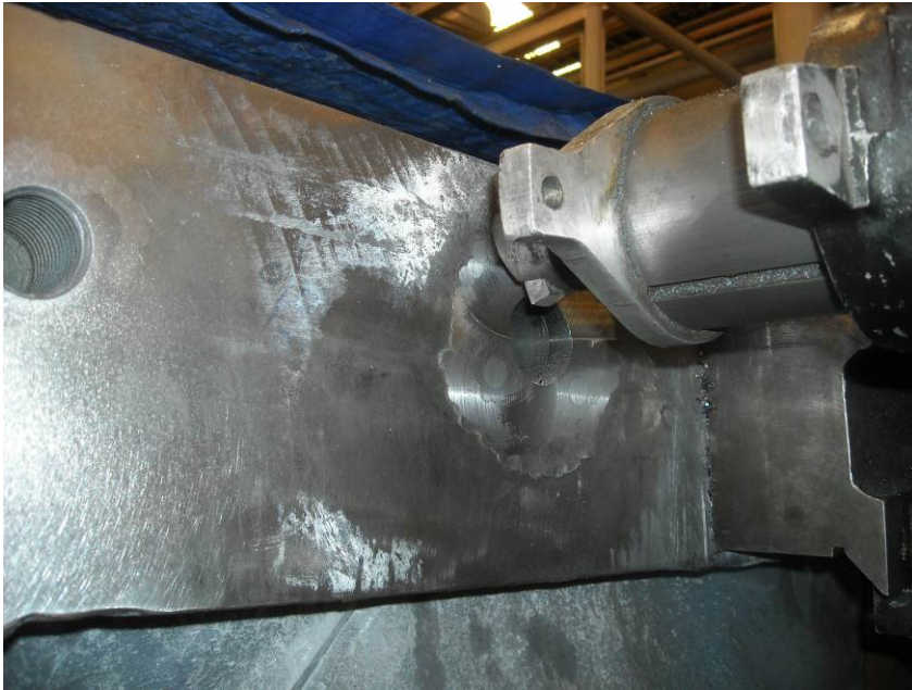
In process of milling of the installed plate.
