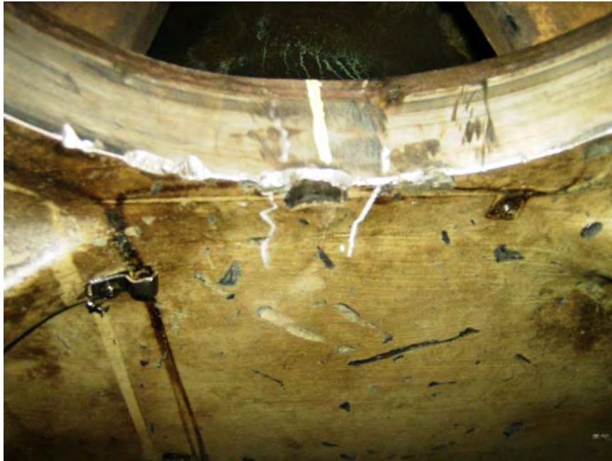
Lower bore damage
