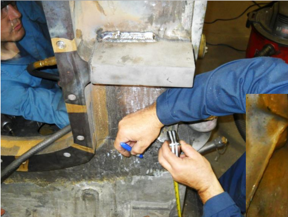
Outer gusset flanges repaired
