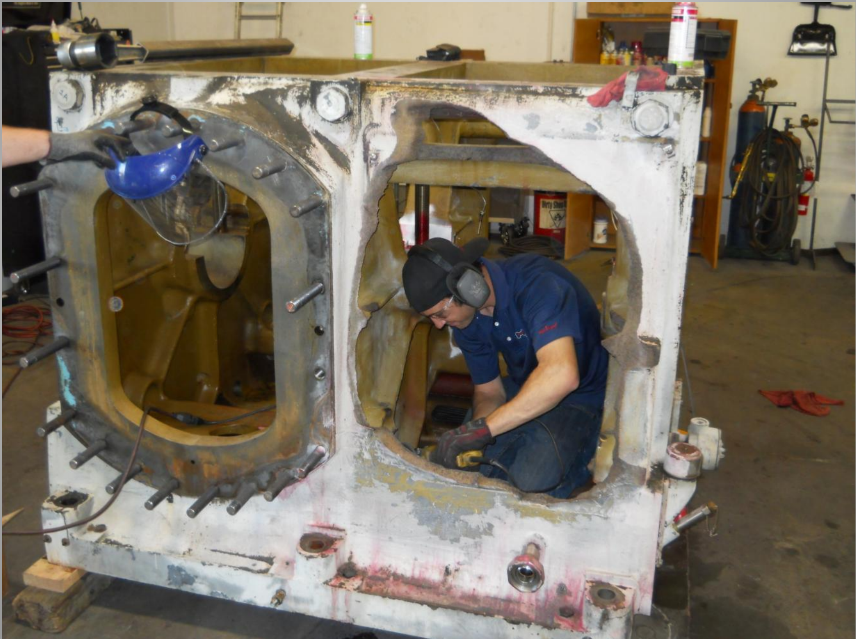
Frame at LOCK-N-STITCH Inc. where the prep work begins on the damaged area
